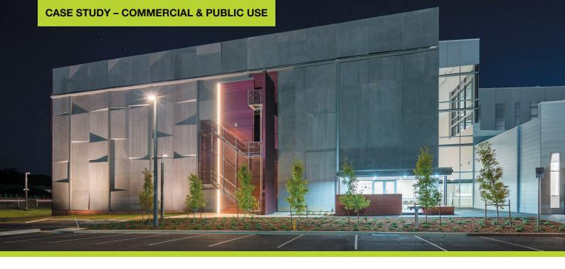
Each measuring approximately six by three metres, the panels are stacked vertically, three to a stack.
